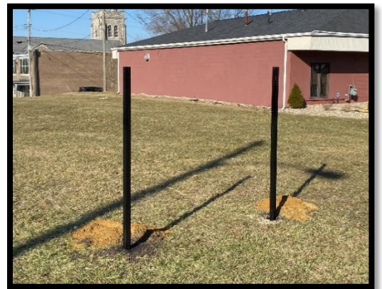
Set posts, sleeves & gravel backfill
