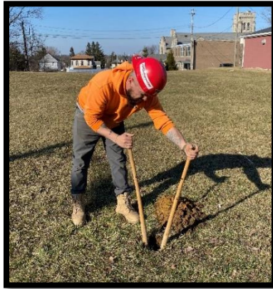
Dig post holes
